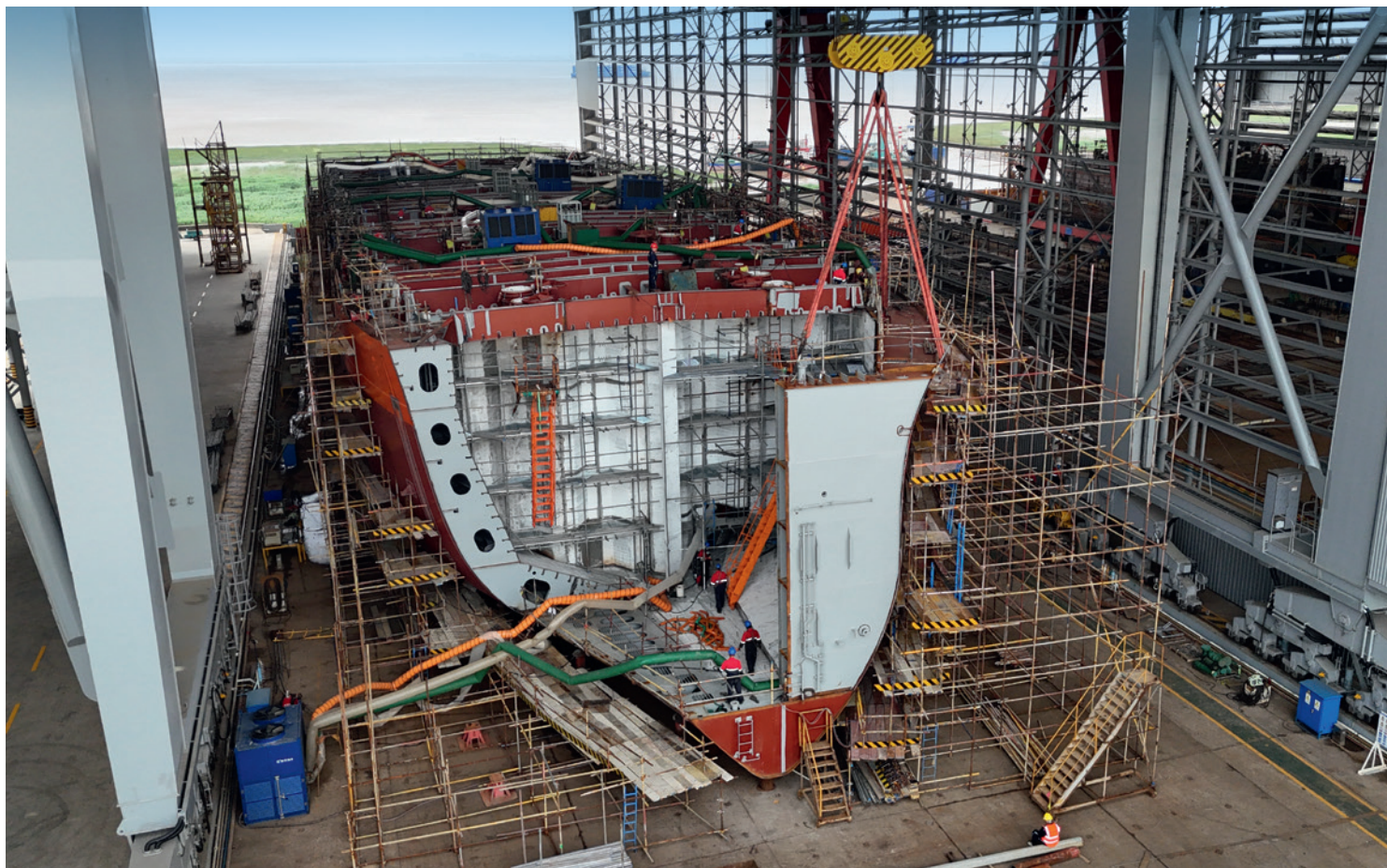
A part of the bow section is lifted and integrated into the tanker structure. In the background the green meadow is visible that still separates the vessel from the Yangtze River. But dredging has begun
